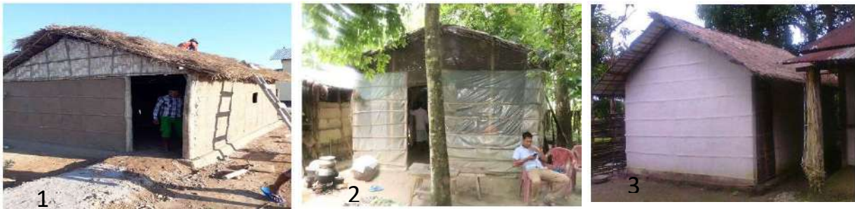
Fig 1-3 (left to right) designs of low cost self cooling mushroom hut designed by TIC
