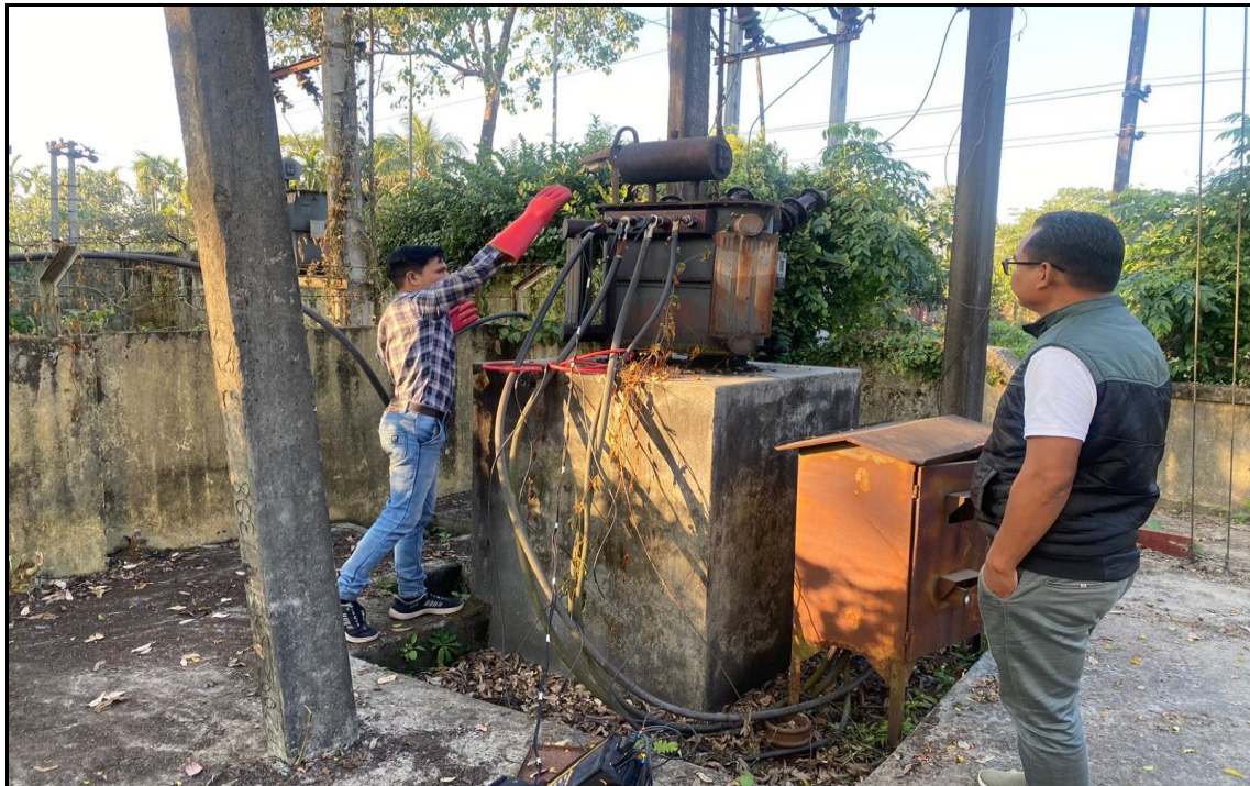
Power Measurement on Transformer
