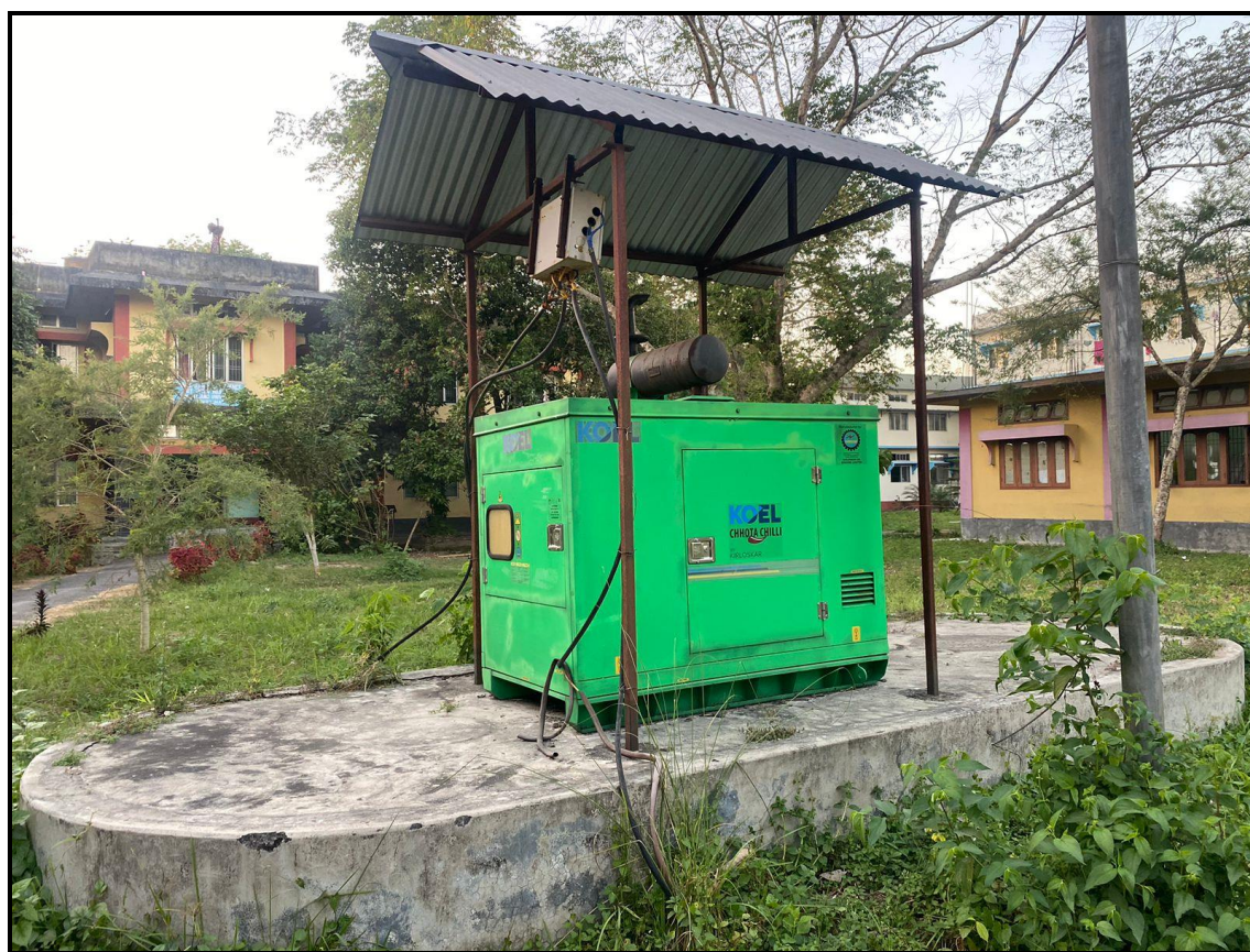
Figure: - DG sets for hostels
